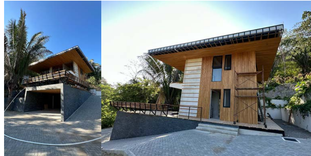
House 1 under construction. Completion date: July 2023.
