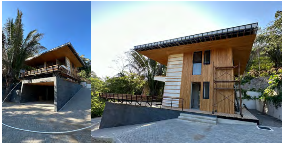
House 1 under construction. Completion date: July 2023.
